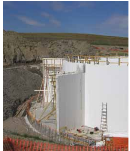
Bioreactor construction at the wastewater treatment plant.
